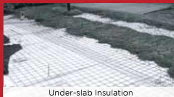
Under-slab Insulation
